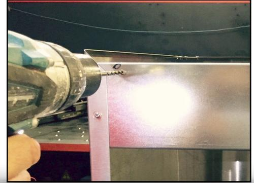
12. Drill holes in back of duct cover at the top.
