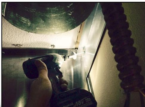
16. Screw duct cover into top plate or blocking using angle drill.
