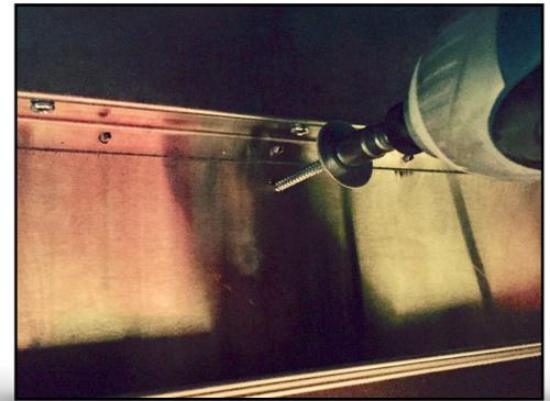
15. Lift hood in to place then install screws in canopy.
