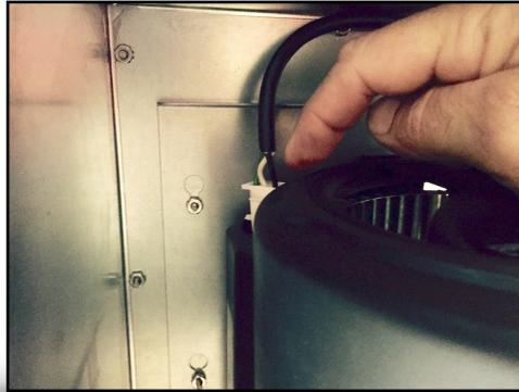
2. Pinch both sides to remove wire connector Qty. 1 600cfm - Qty 2 1200cfm
