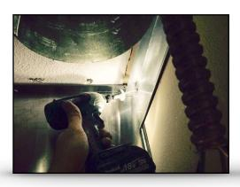
16. Screw duct cover into top plate or blocking using angle. drill.
