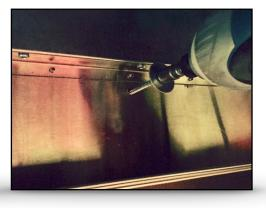
15. Lift hood in to place then install screws in canopy.
