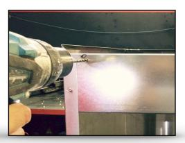
12. Drill holes in back of duct cover at the top.
