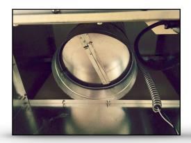
19. Slide duct up into place through bottom of canopy.
