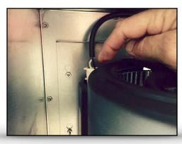
Pinch both sides to remove wire connector Qty. 1 600cfm -Qty 2 1200cfm
